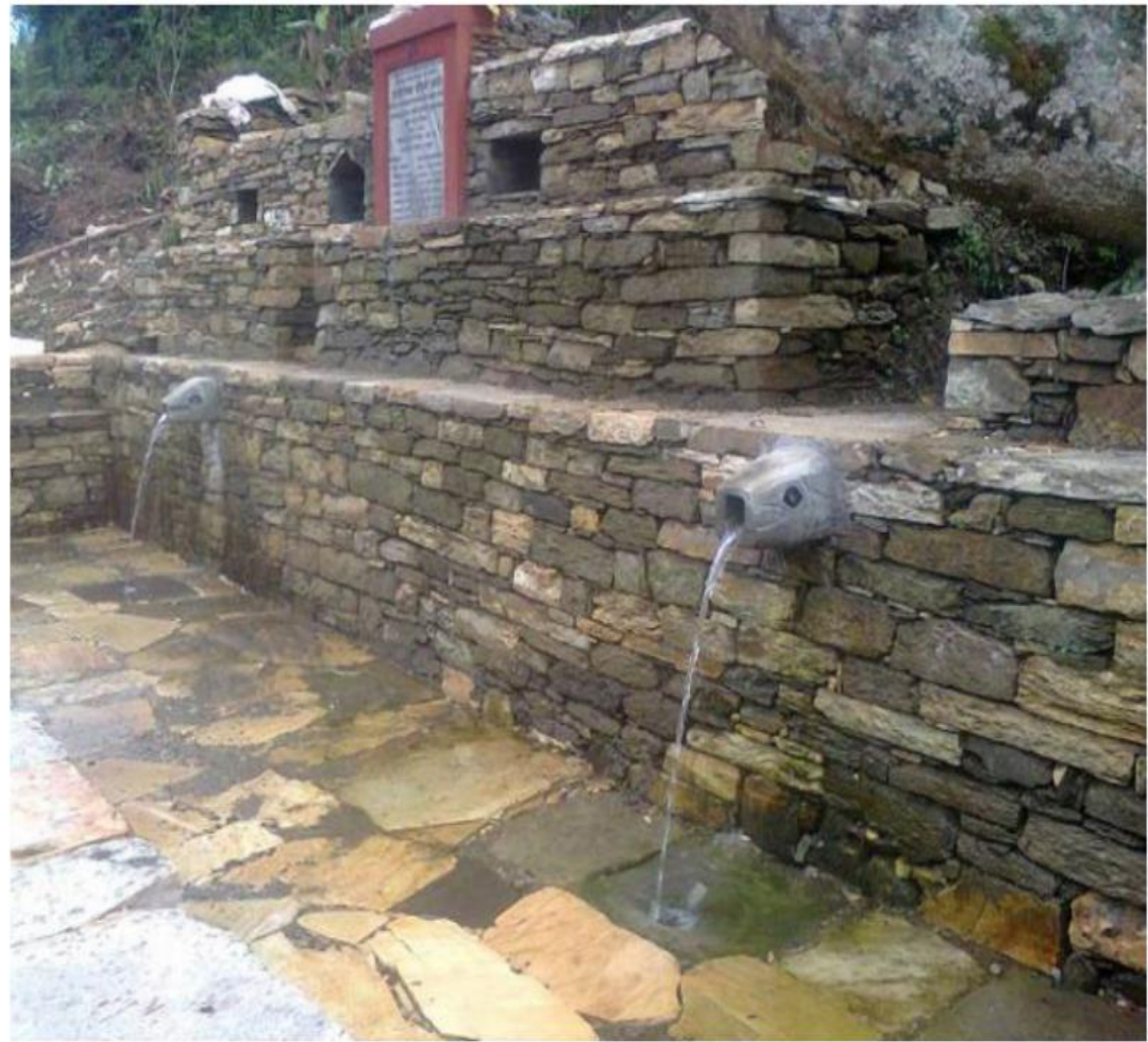
Water Spout after renovation
