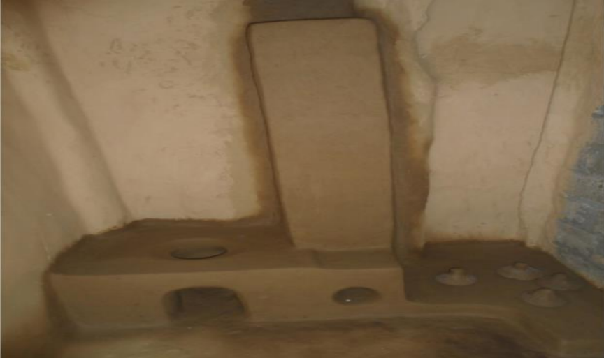
Newly constructed ICS from Trained stove master
