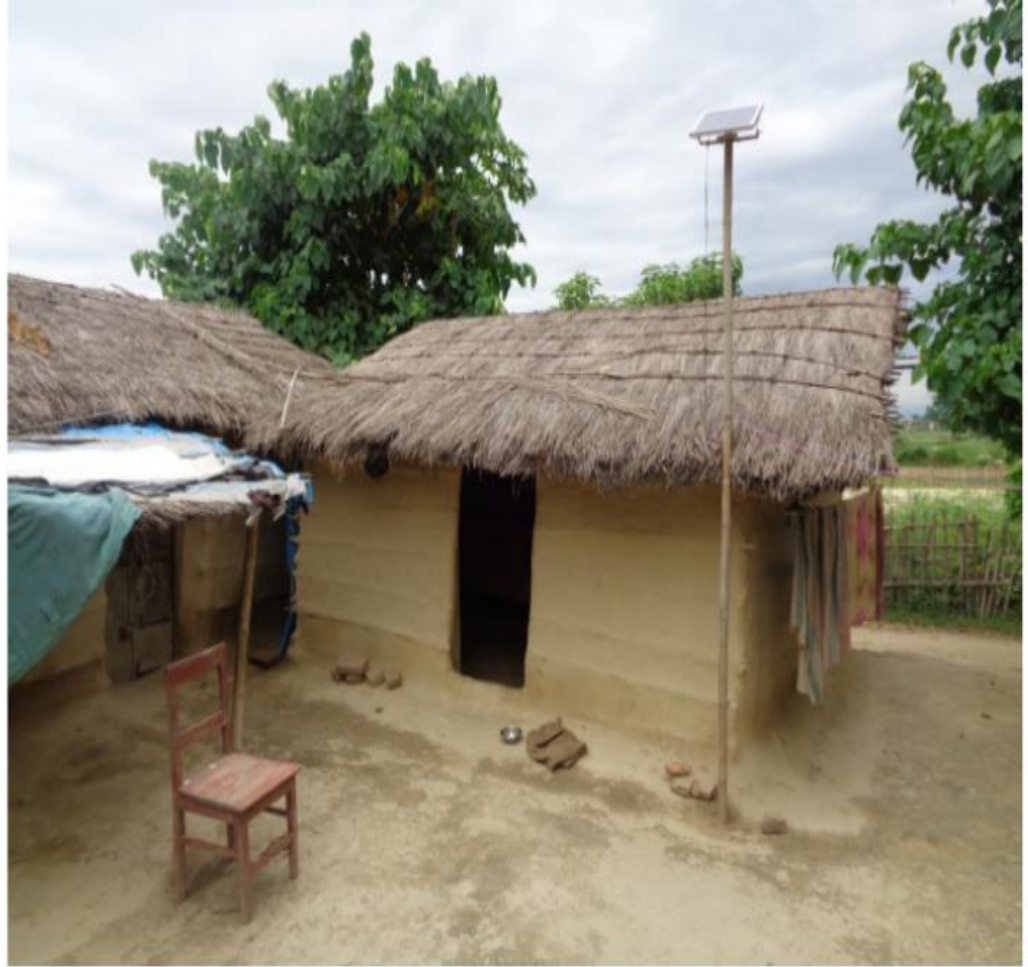
Solar tuki in Kanakpur VDC
